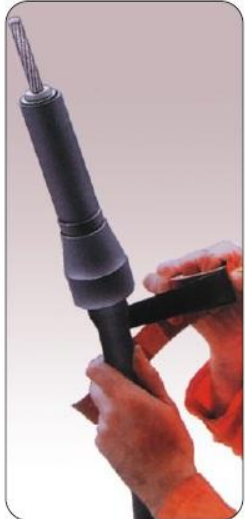
Application of Self Amalgamating Insulating Tape over Stress Grading Pad
