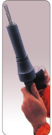
Application on Stress Grading Pad over stress cone and cable outer screen
